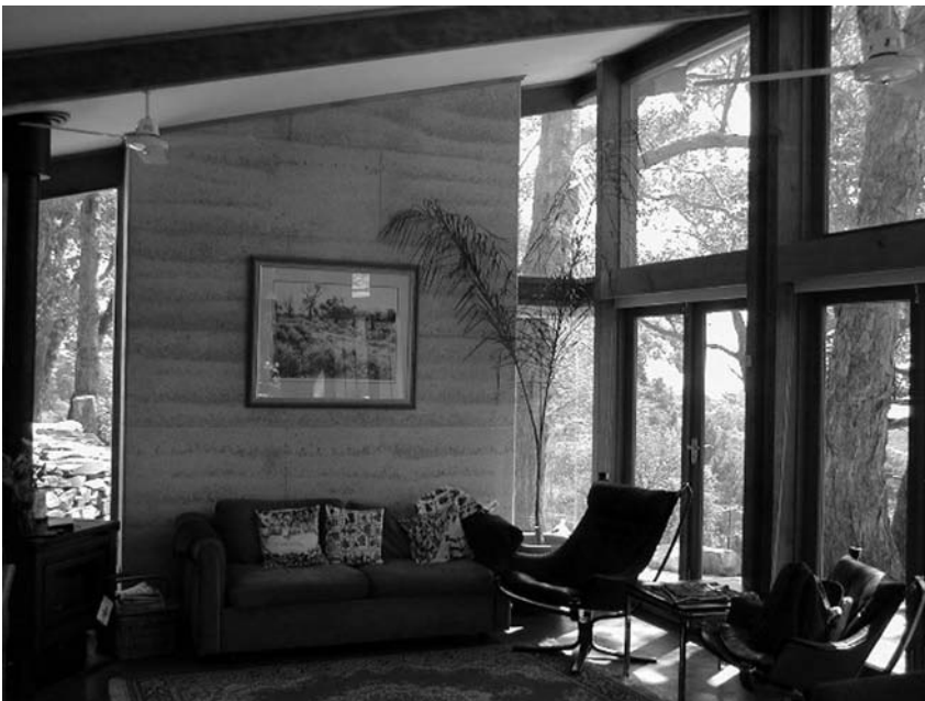
4.25 Living room with rammed earth wall in Kawanda Muna house: the high window can be opened for ventilation
