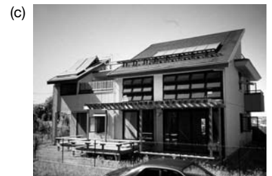
0.8 (a) Akamine residence, Japan: the storage wall is made of coral stones; (b) TMU house I, Japan: water flows onto the roof creating a thin film which evaporates enhancing cooling of the roof; (c) 'Echos I', Japan, has a flat plate collector for hot water supply (left roof) and a crystal-type photovoltaic panel (right roof)
