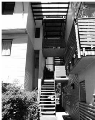
7.22 Cotton Tree Housing: permeable stairways in the three storey units facilitate airflow across the site
