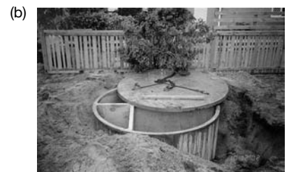
Figure 9.35 Prosser House: grey water system
