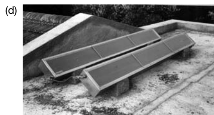
10.11 Casa Solar project shows the integration of a solar system with other passive elements of the building: (a) a renovated farm building is earth integrated; (b) an external pergola is provided to give an external living area; (c) the pergola has integrated PV solar systems; (d) the roof is used for solar thermal hot-water heating
