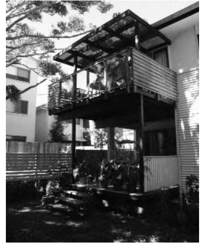
7.27 Cotton Tree Housing: external rooms are constructed of a lightweight elemental system (bolt on and off) for ease of maintenance
