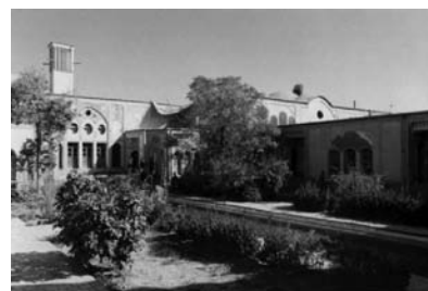
5.17 Rooftop of the summer residence showing the wind catchers
